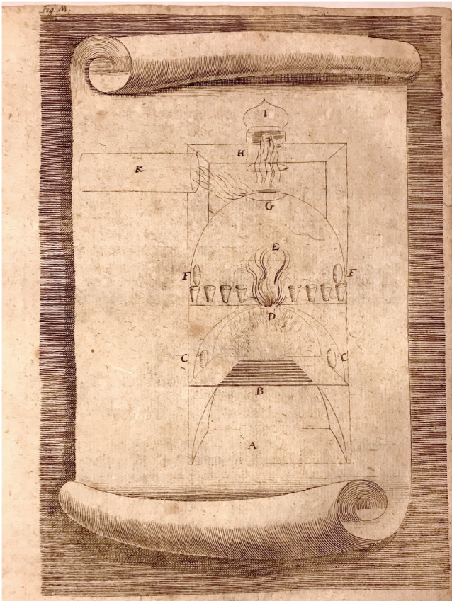
FIGURE 2 Sketch of Kunckel's compendious furnace that contains several small crucibles used for testing (F). Especially noteworthy is the fire channel (K) that could be used to hook up another and smaller furnace. 9 Source: Photo © Thijs Hagendijk
